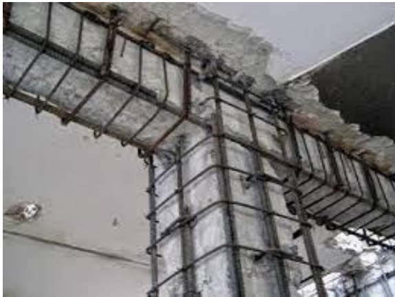
Column Beam Joint Jacketing
