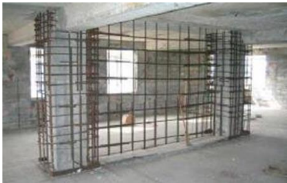
Adding Shear Wall
