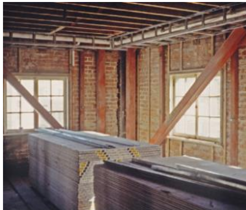
Adding Shear Wall
