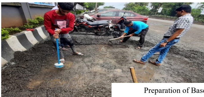
Initial Site condition & removal of loose materials
