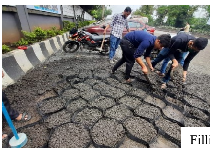
Figure 2: Sequence of road shoulder stabilisation using geo-cell
