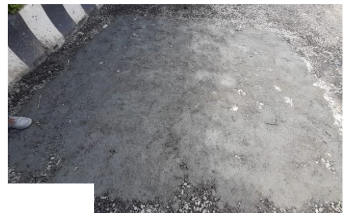
Filling, compacting & surface finishing of shoulder
