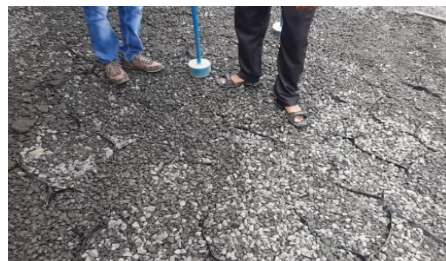
Filling, compacting & surface finishing of shoulder
