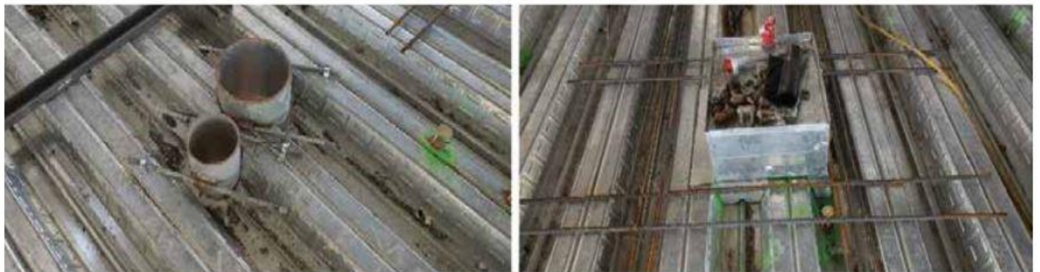
Figure 2. Schematic configuration of sleeving and boxing-out openings.
