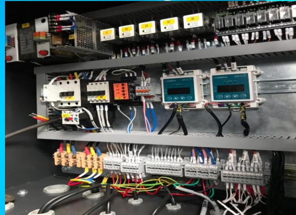
Control panel for compressor
